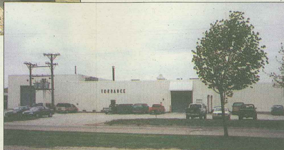
The Rock Island office (above) along with the existing operations in Cedar Rapids, Waterloo, Des Moines, Mason City, Dubuque and Iowa City, are positioned to continue providing companies the lift truck equipment and services needed for their success into the next millennium.
